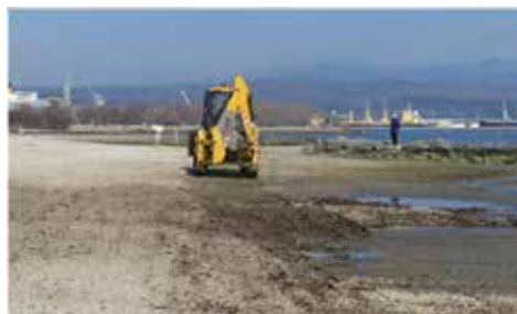
Excavator combs beach on the Adriatic Sea
